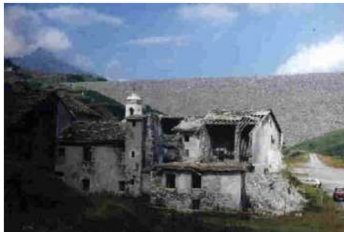
The village of Grand Croix, the only surviving settlement on the Mont Cenis. In the background is the wall of the reservoir. - Photo: PG.
